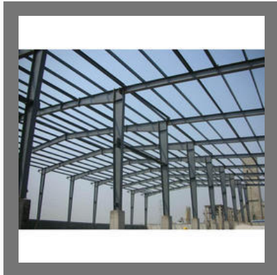
Steel Industry Structure Fabrication Service
